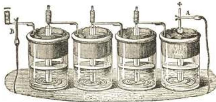
FIG. 43. GRAVITY BATTERY OF THE TROUVÉ-CALLAUD TYPE.
